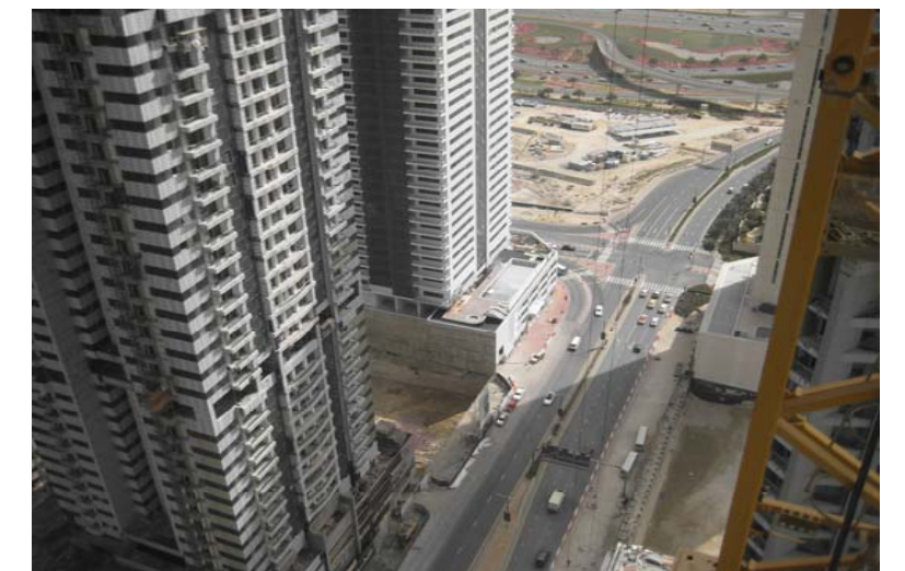
Road going towards Marina Mall
