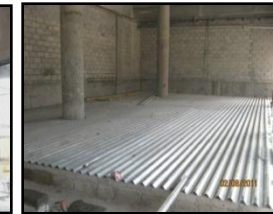
GF Slab high level
