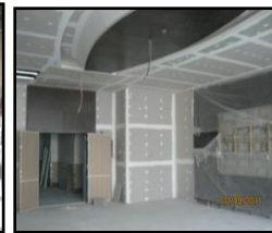
5 th Floor joinery works
