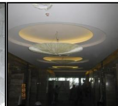
5 th Floor Gypsum Board and Light Fitting
