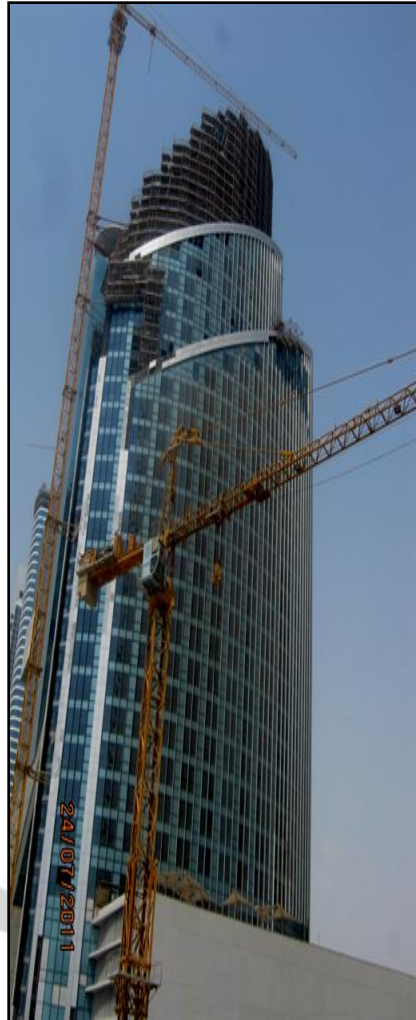
External Façade showing the progress of Cladding
