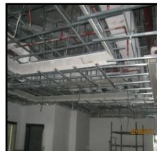
5 th Corridor False Ceiling
