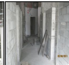
5 th Floor Cafeteria
