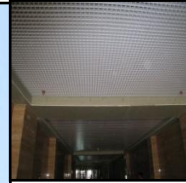
false ceiling @ GF
