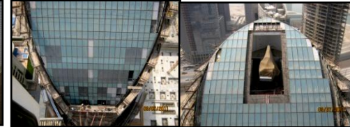
Upper roof external cladding progress
