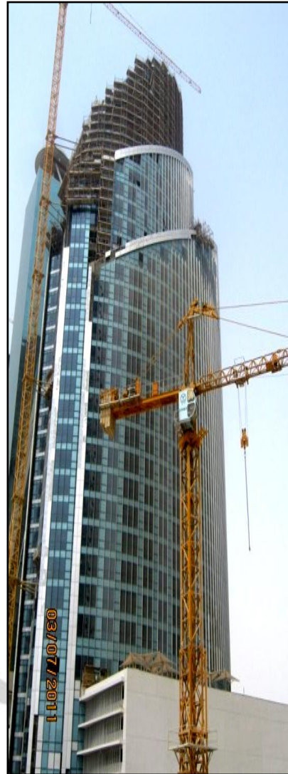
External Façade showing the progress of Cladding
