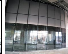
Cladding Works in GF Retail & main Cafeteria
