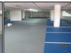
Epoxy Flooring at Parking Area
