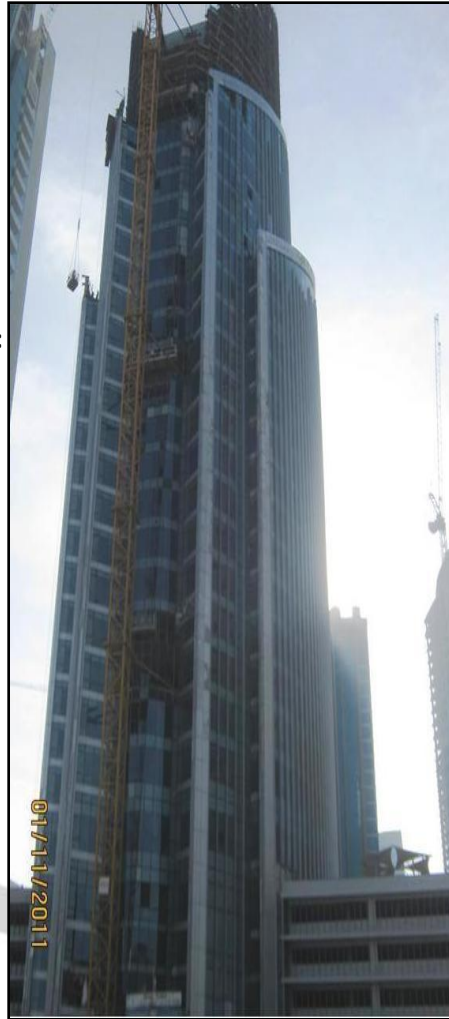
External Façade showing the progress of Cladding
