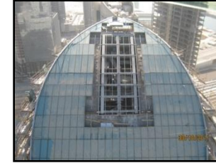
Upper roof external cladding progress
