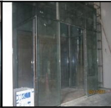
GF Glass Door & Frame fixing for Air lock
