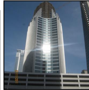
Backside Elevation cladding
