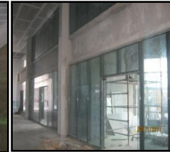
GF Glass Door & Frame fixing for Air lock
