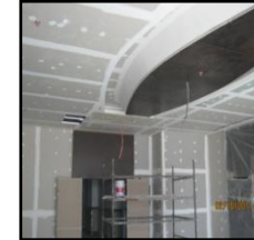
5th floor joinery works
