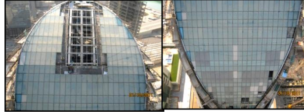
Upper roof external cladding progress
