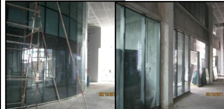
Cladding Works in GF Retail & Main Cafeteria
