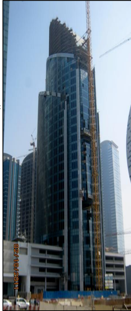
External Façade showing the progress of Cladding
