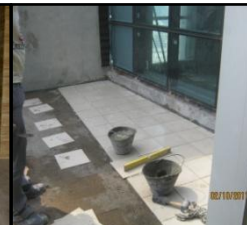
Ceramic fixing for Balcony area at 24th floor
