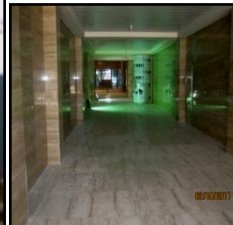
GF back entrance False Ceiling
