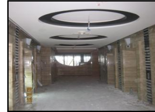
5th floor Wood Fixing for Lift lobby Corridor
