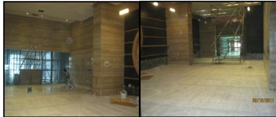
GF joinery work progress at the Reception Hall
