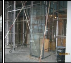
GF Frame fixing for Air lock
