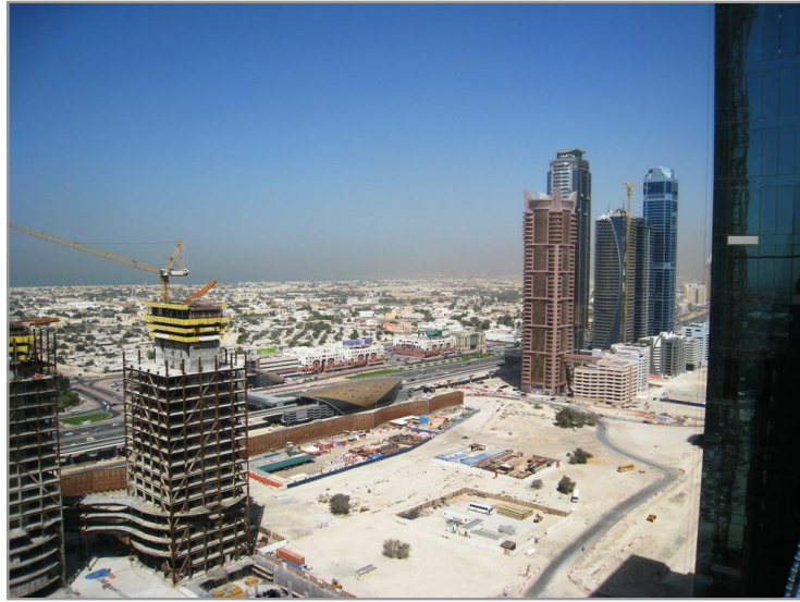
LOOKING EAST SIDE OF SHK. ZAYED ROAD
