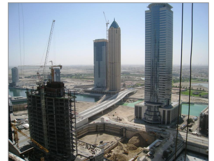
LOOKING AT NEIGHBORS TOWERS & PARTIAL VIEW OF CANAL
