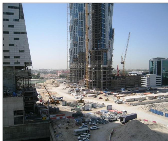
LOOKING WEST SIDE OF SHK. ZAYED ROAD
