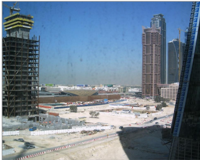
LOOKING EAST SIDE OF SHK. ZAYED ROAD
