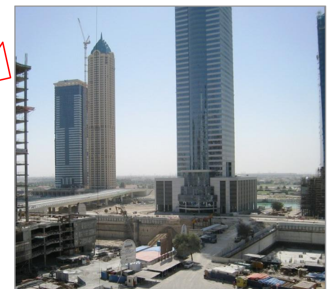
LOOKING AT NEIGHBORS TOWERS & PARTIAL VIEW OF CANAL
