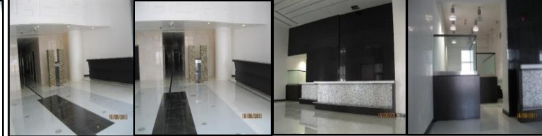
Progress of Works on Ground Floor Reception Hall & Cafeteria
