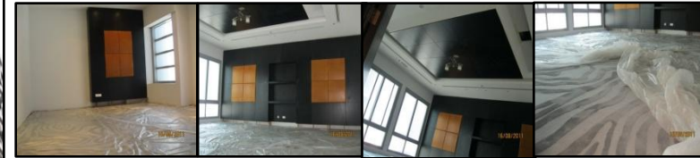
Progress of Fit Out Works on 5th Floor Meeting Room
