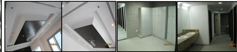
Progress of False Ceiling @ Meeting Rooms Gymnasium Lockers & Lavatory
