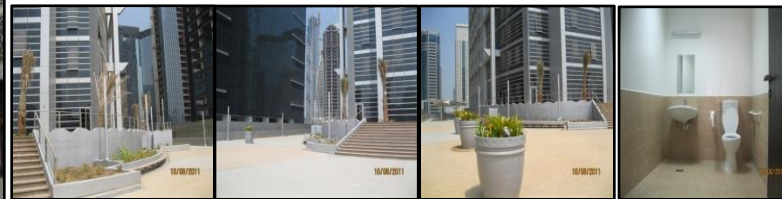
5th Floor Podium & Landscaping are 100% completed
