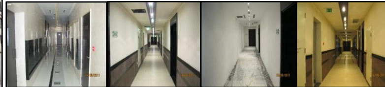
GF and 5th Floor Hallway Fit Out are 100% completed
