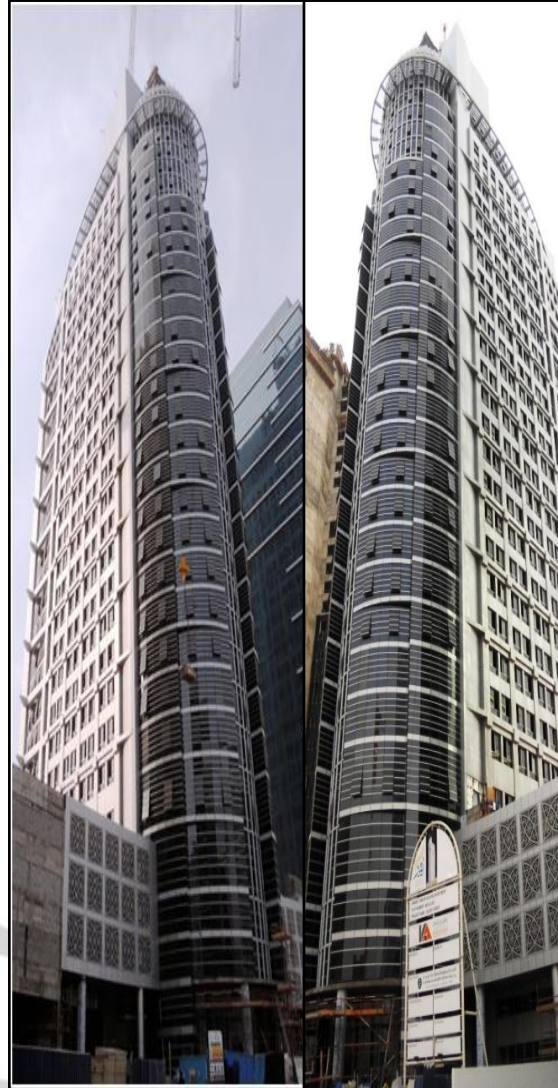
Front, Back & Sides Elevations Cladding Works 100% Completed
