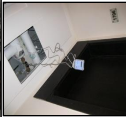
Installation of BTU Meter
