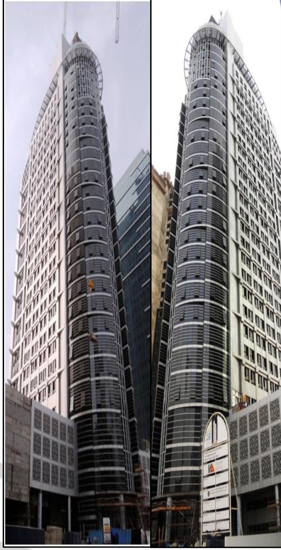
Front, Back & Sides Elevations Cladding Works 100% Completed
