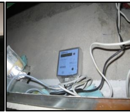
Installation of BTU Meter
