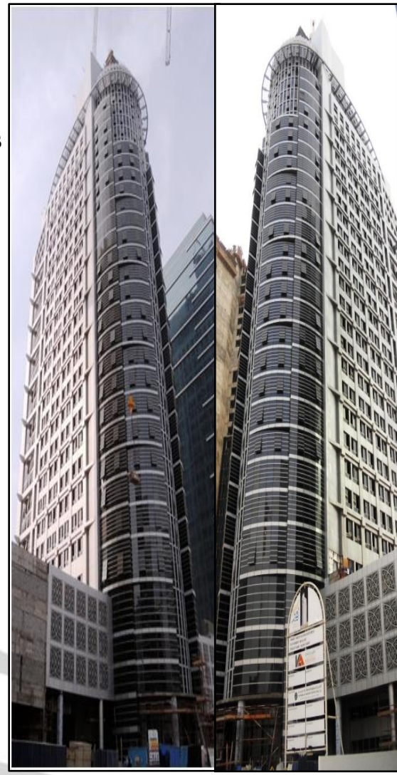
Front, Back & Sides Elevations Cladding Works 100% Completed
