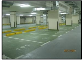
Road Marking, Numbering and Installation of Wall Guard at Parking Area
