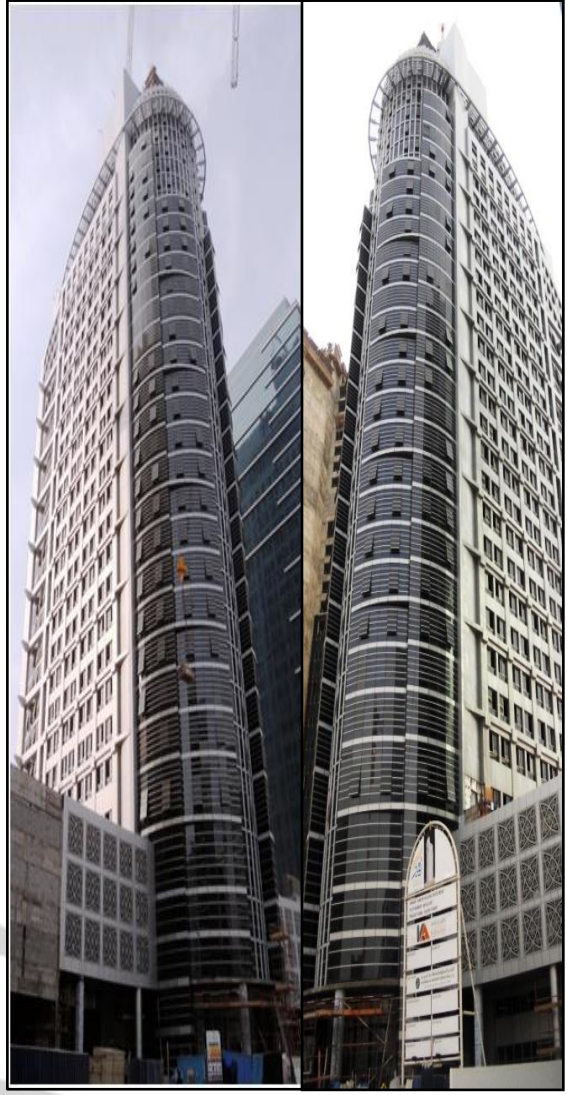
Front, Back & Sides Elevations Cladding Works 100% Completed
