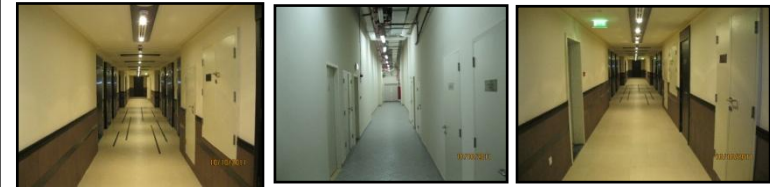
GF and 5 th Floor Hallway Fit Out are 100% completed
