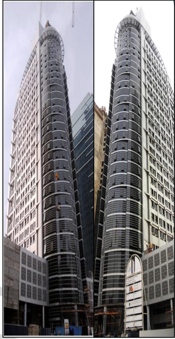
Front, Back & Sides Elevations Cladding Works 100% Completed
