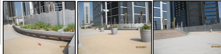
Hardscape work at podium level
